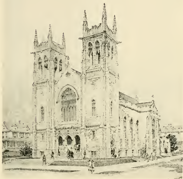
FIG. 92. — HOLY SPIRIT CHURCH, Atlantic City. In course of construction.
